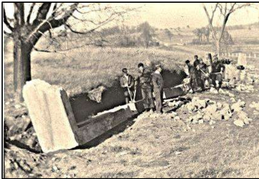
CCC workers removing a non-historic foundation at Saratoga National Historical Park
